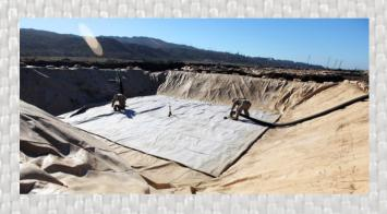
AEF highly recommends a secondary containment for all fuel tanks for added protection. We can provide customized berm liners to meet your applications.
